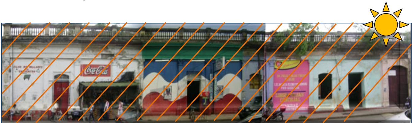
Vista Principal Sureste (Incidencia Solar)
