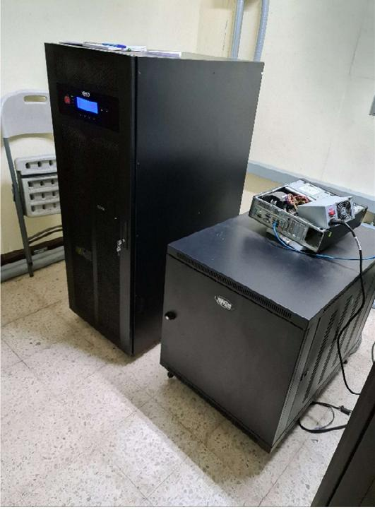
A black Tripp Lite SUT20K UPS unit is shown in a room. It is a tall, vertical cabinet with a digital display on the front. A smaller, silver-colored component is placed on top of the unit. The unit is on a tiled floor. | <p><b>1. UPS TRIPP. LITE 20KVA</b></p> <p>UPS marca TRIPP. LITE de 20KVA, 208VAC 3 Fases + Neutro</p> <p>Modelo SUT20K</p> <p>Equipo moderno en óptimas condiciones</p>  |
