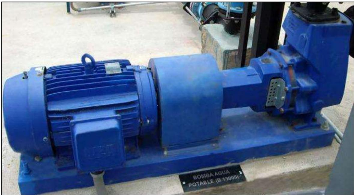
*Figura No. 9: Bomba de agua potable instalada en Biwater.*
